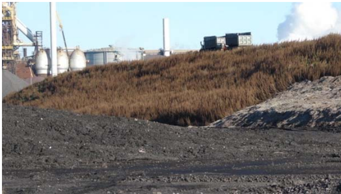
Construction of Berm along south side of coal field
