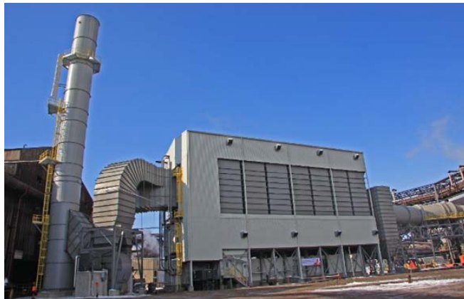
#7 Blast Furnace Baghouse
